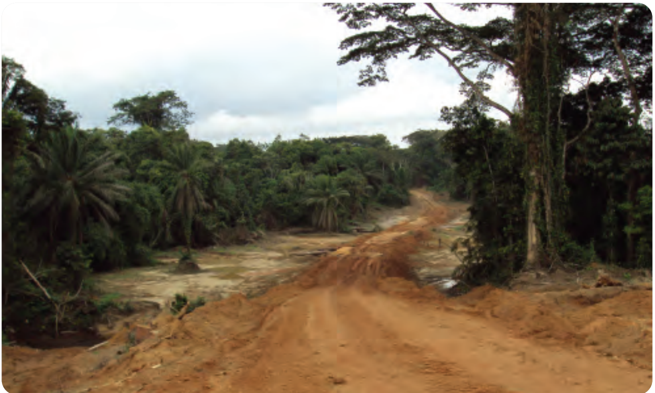
Logging access roads lead to conversion of the natural forest to other land uses. Photo: SDI
