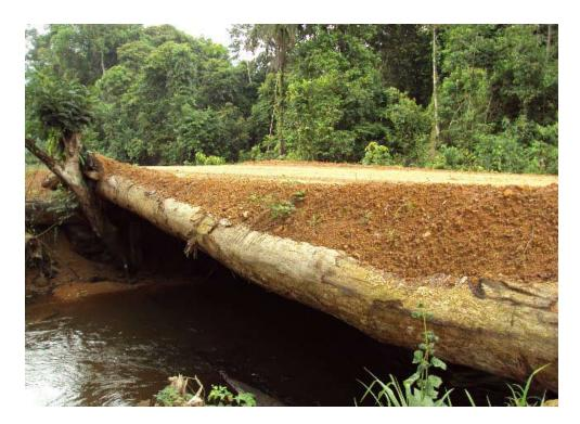
I Log bridge constructed by Tarpeh Timber. Although the company stated that it would not construct log bridges on major roads in the area; that is exactly what it has done.
